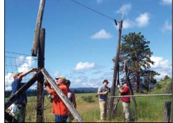
OHA members work to repair the fence at White River Wildlife Area.
